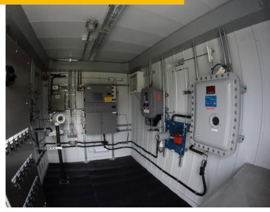
The Gulf South FERC NGA Gas Tariff specifications for the Coastal Bend Header stated the receipt stations must have on-line monitoring equipment installed at each interconnect detecting oxygen, moisture, hydrogen sulfide (H<sub>2</sub>S), BTEX components (benzene, toluene, ethyl-benzene, and xylenes), and mercury (Hg). The equipment needs to detect deviations from established Gas Quality Standards in real time, to allow the interception of such gas from the Coastal Bend Header.
